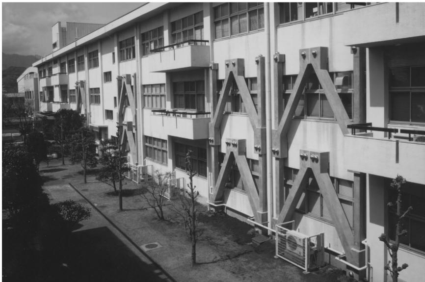
**Fig.1 photo of installed PCa brace on peripheral frame**
