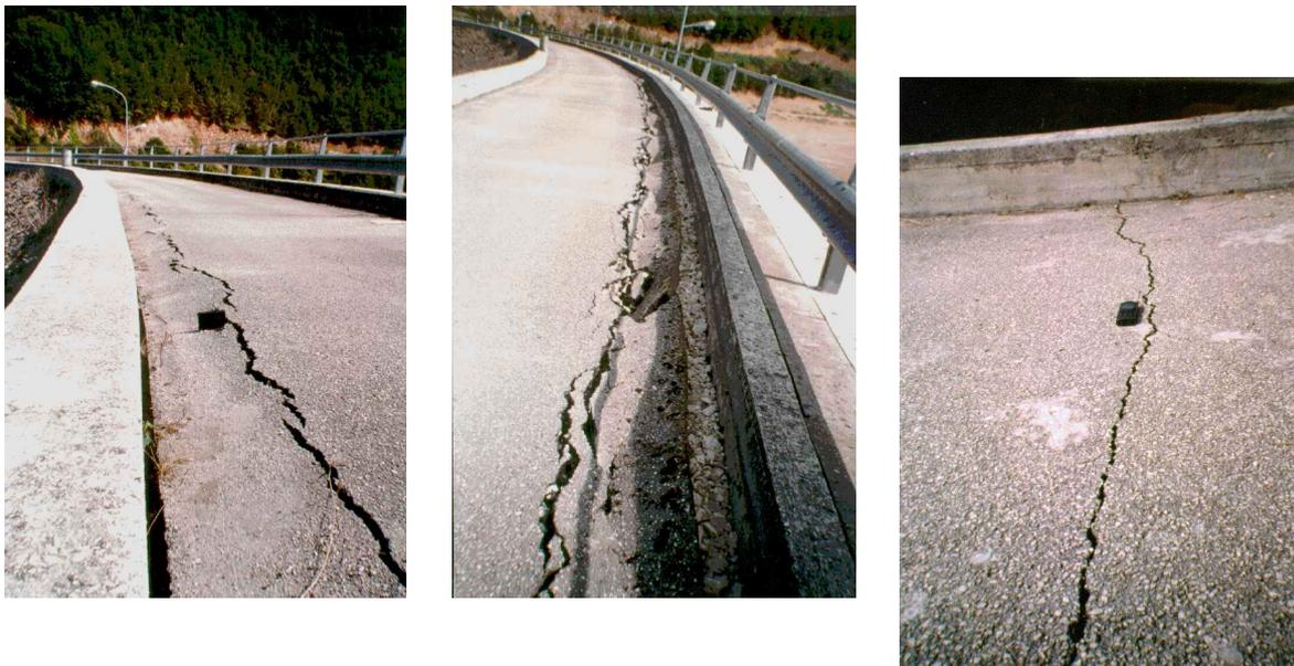
**Figure 5: Damages of Acciano (Perugia, Italy) earth dam.**
