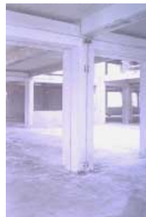
Fig. 15. Prefabricated building in construction (R-4)
