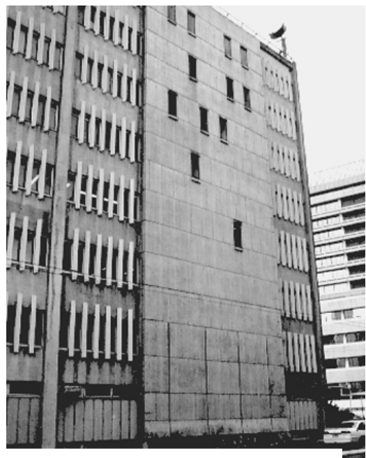
Figure 9: Reduced fenestration towards wall base, Wellington Central Telephone Exchange
