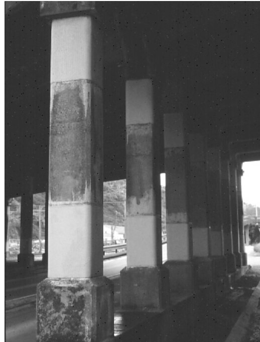
Figure 6: Wrapped potential plastic hinge regions
