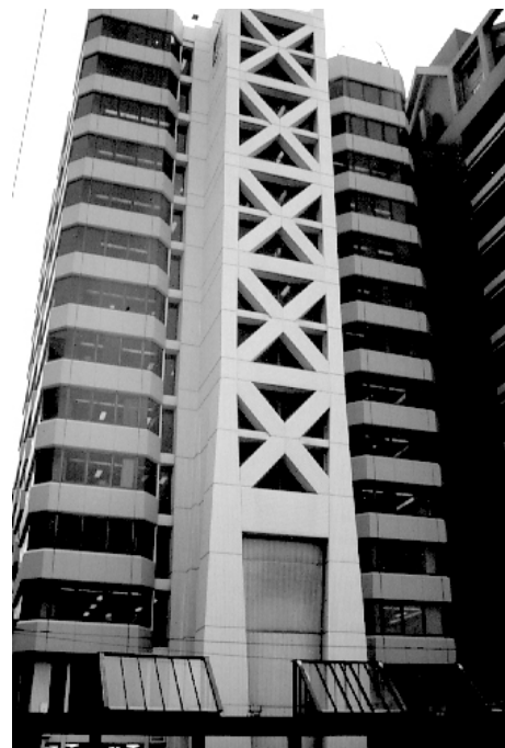
Figure 2: Cross-braced tower, Wool House, Wellington
