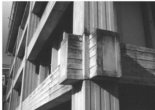
Figure 7: Typical beam stubs
