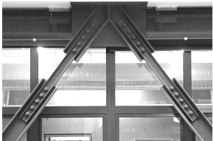
Figure 8: ‘Fuses’ in cross-bracing, Schools of Architecture and Design, Wellington
