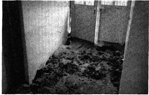
Figure 3. Sand boil from a room floor in Astaneh.
