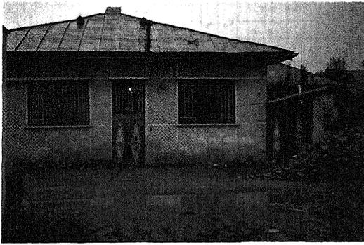
Figure 5. Liquefaction induced differential settlement between a house and its adjacent wall in Astaneh.
