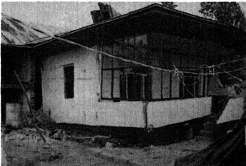
Figure 2. Extent of liquefaction induced damage to a house in Astaneh.
