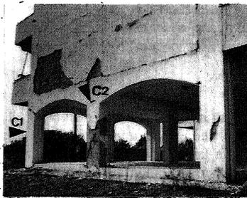
Figure 2. Damage of the ground floor structural elements and of the first story masonry infills (view from column C2 see also fig.1).
