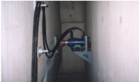
Photo. 5 Static Loading Test By Using Oil Jack
