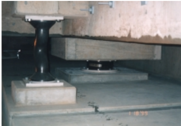
Photo. 3 Base Isolation Devices
