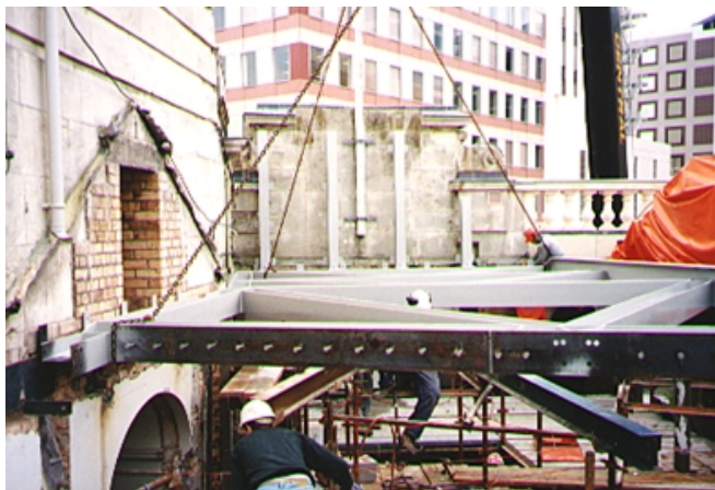
Figure 9: Tower Restraint Truss
