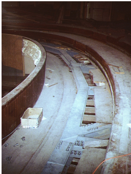
Figure 8: Circle Truss Inner Chord within Circle Bleachers
