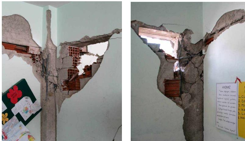
**Figure 8. Shear failure of captive columns as a result of crushing of upper corner of masonry walls in building C-14-01.**
