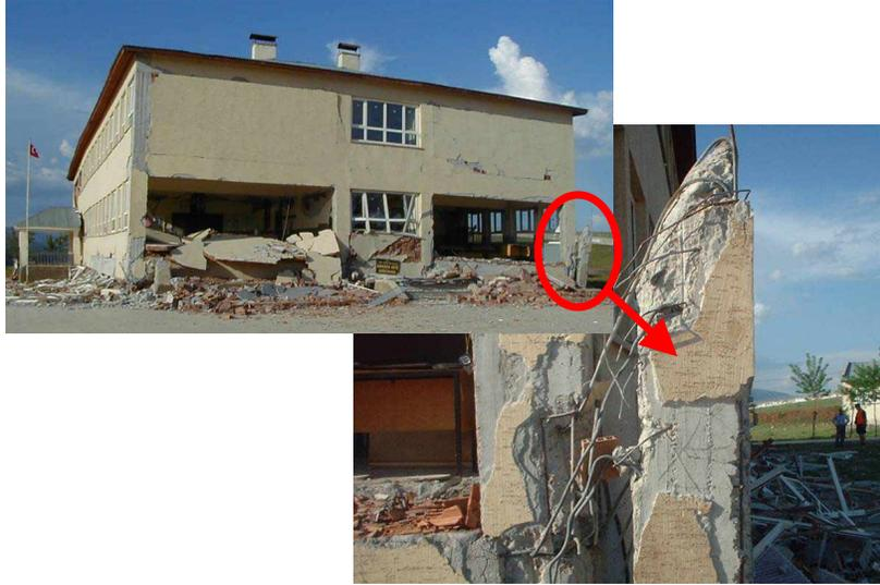
**Figure 9. The shear failure of the corner column in building C-13-09 (collapsed). The spacing of the transverse reinforcement is 10 cm at the top 30-cm portion of the columns. The ends of the stirrups were not anchored properly.**
