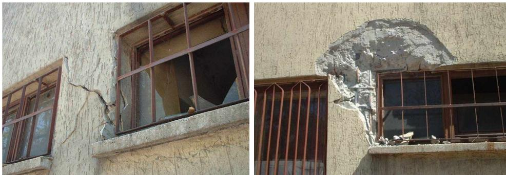
**Figure 7. Shear failure of captive columns created by the small windows of the furnace room in building C-14-03.**
