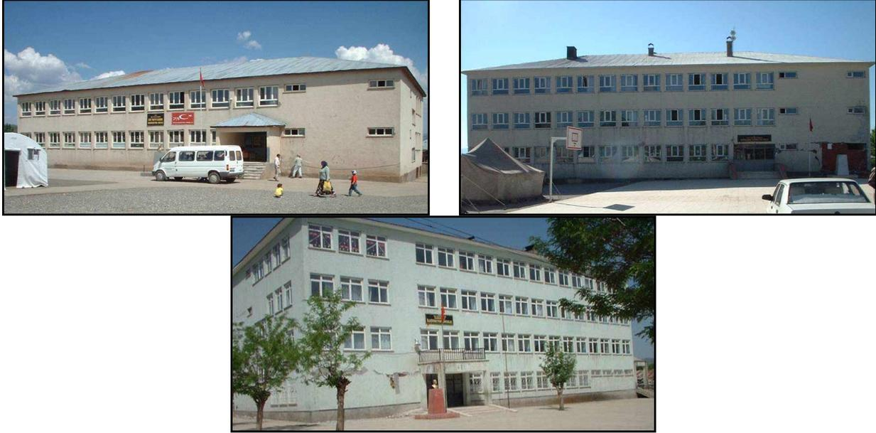
**Figure 5. School buildings with typical floor plan without shear walls**
