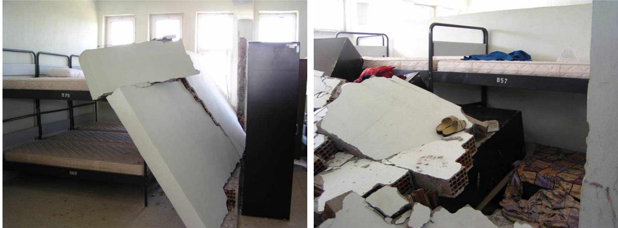
**Figure 15. Collapse of the free standing masonry walls onto the beds in the dormitory buildings.**
