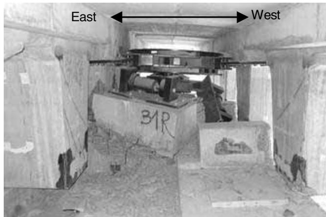
**Figure 6. The damage caused by the relative movements of the girders with respect to the piers**
