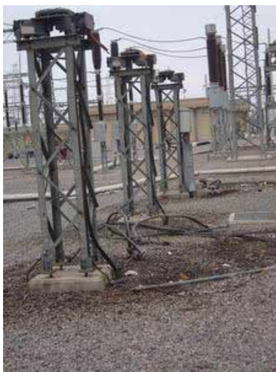
(Fig-2)- Equipments was broken at connection joint between electrical components and fitting which was connected themes to support box and structural part
