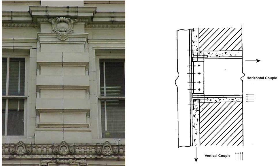
Figure 7. Typical exterior column and masonry infill; schematic depiction of horizontal and vertical resisting couples for beam-column connection.
