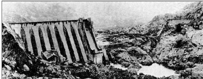
Fig. 2 Vega de Tera Dam after collapse
