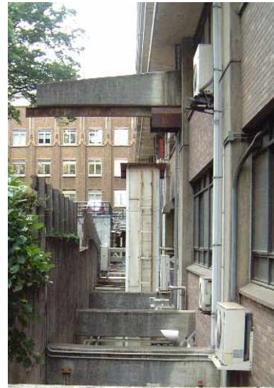
Figure 2 Dry area and flying beams on south elevation before retrofit (view from east to west)
