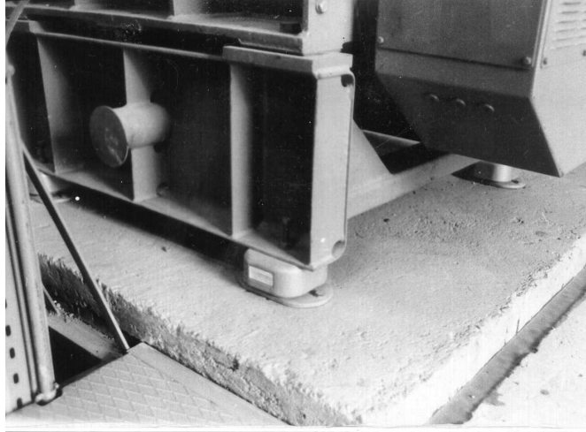
Figure 7: Power generator vibration isolators
