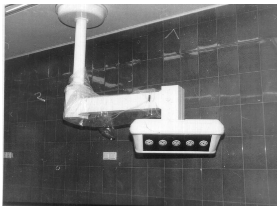
Figure 10: The medical gas panel in surgery room
