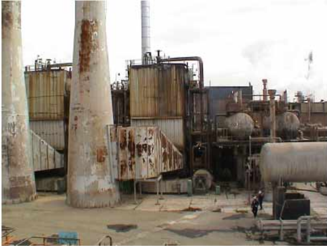
Figure 5: Boilers produce steam for all steam turbine drivers and other refinery needs
