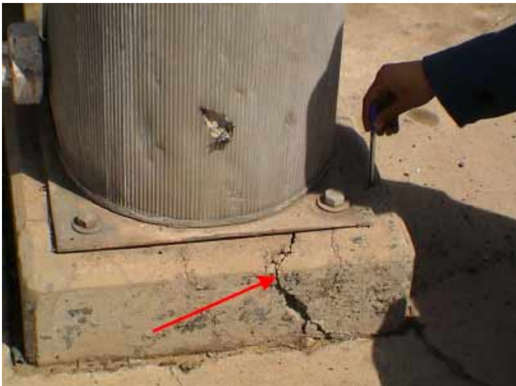
Figure 6: Deep cracks in foundation
