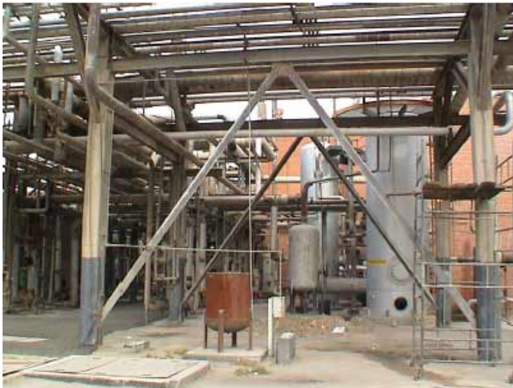
Figure 8: Bracings of the pipe supporting system
