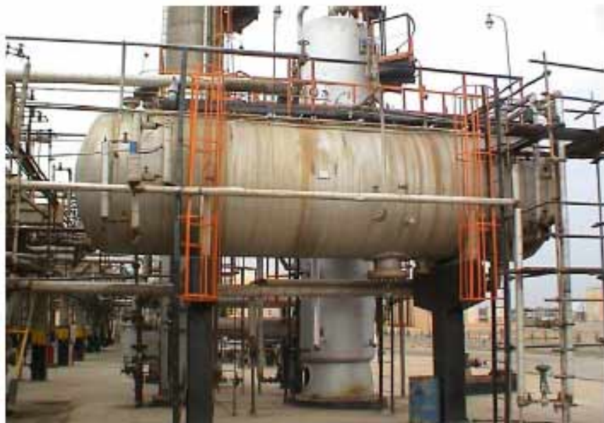
Figure 4: Surge drum in old sour water stripper unit
