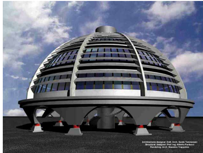
Figure 5. The isolated "dome building" of the Emergency Management Centre in Foligno (Italy)
