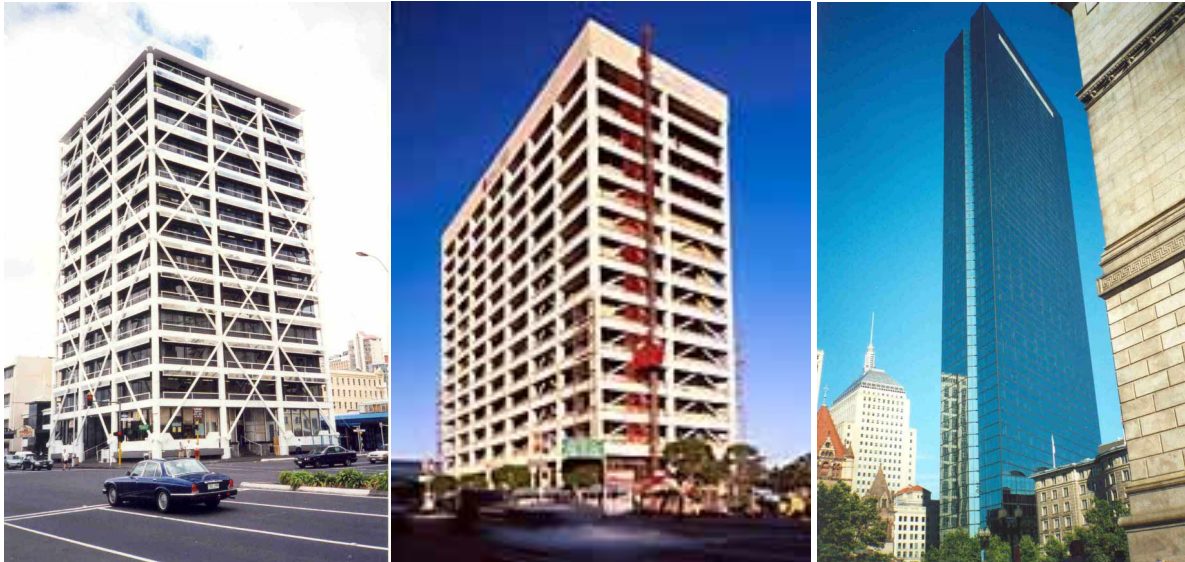
Figure 1. Buildings with innovative systems: Union House, Auckland (base isolated); Cal Fed Building, Sherman Oaks (friction damper braced); John Hancock Tower, Boston (hybrid control equipped)
