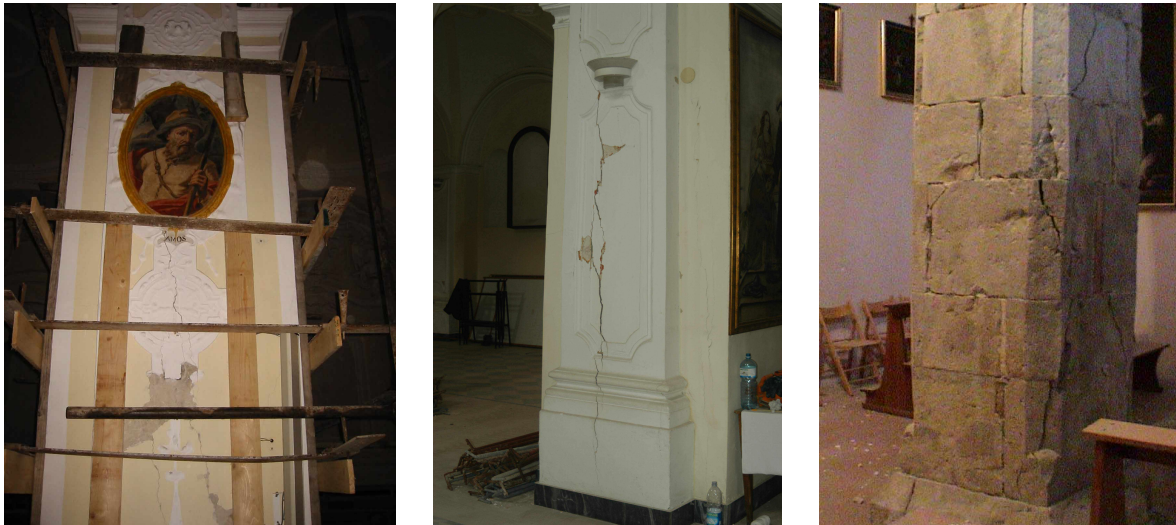
Figure 5. - Three examples of crushing damage in masonry pillars
