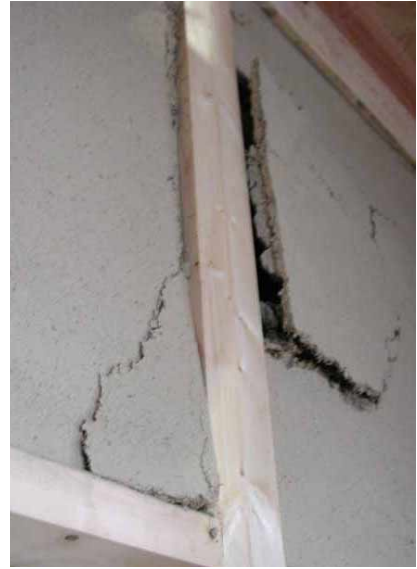
Fig.7 Separation of mud-walls from frame.
