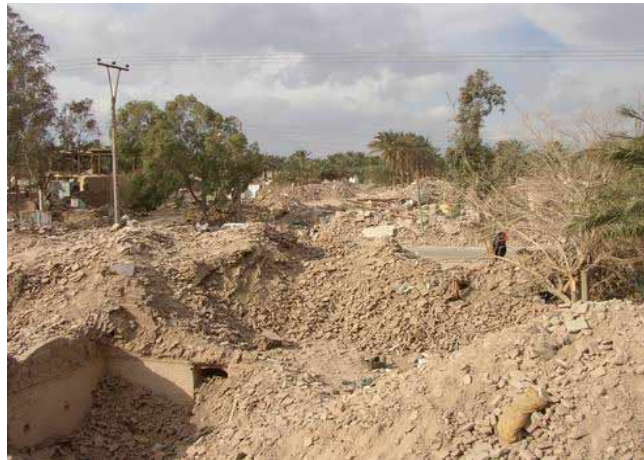
Fig. 6: ground shaking was so severe that the abode houses were turned into their original sun-dried bricks in the Bam 26.12.2003 earthquake.
