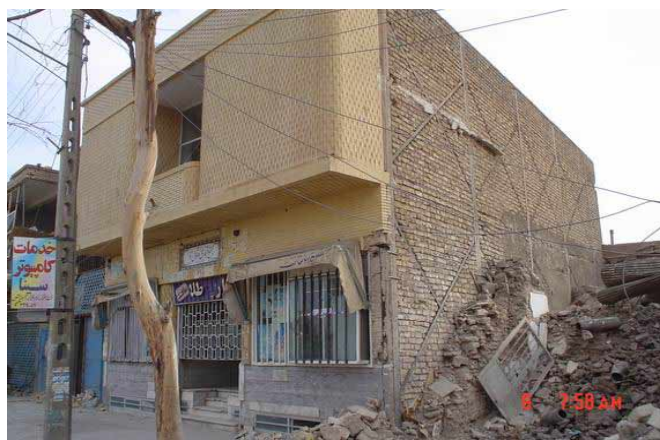
Fig. 11: steel building with good performance during the Bam 26.12.2003 earthquake
