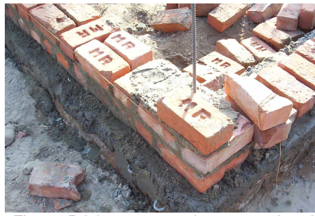
Fig. 8. Brick masonry using rat-trap bond and English bond
