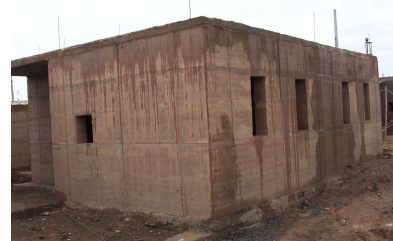
Fig. 11. Stabilized rammed earth house with RC slab roof
