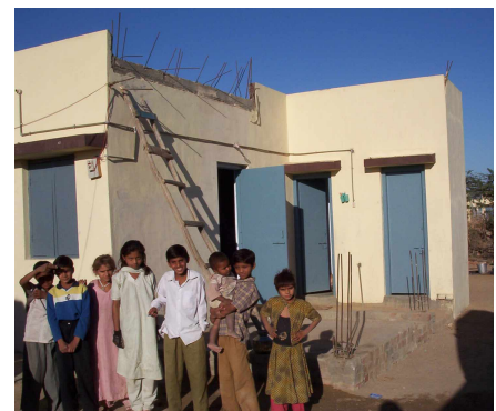
Fig. 13. Flat roofed house with preparations for second story
