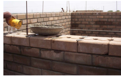
Fig. 10. Interlocking compressed stabilized earth wall
