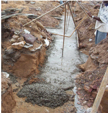
Fig. 2. Unreinforced concrete base layer for strip footing, with vertical steel bars
