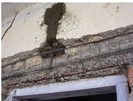
Fig. 14. Wire mesh and tie-rods for ferrocement belt at lintel level
