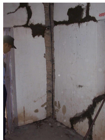
Fig. 15. Vertical bar with shear connectors
