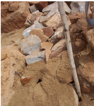
Fig. 4. Random cobble foundation covered with loose sand
