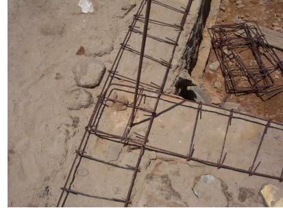
Fig. 6. Reinforcement for plinth band
