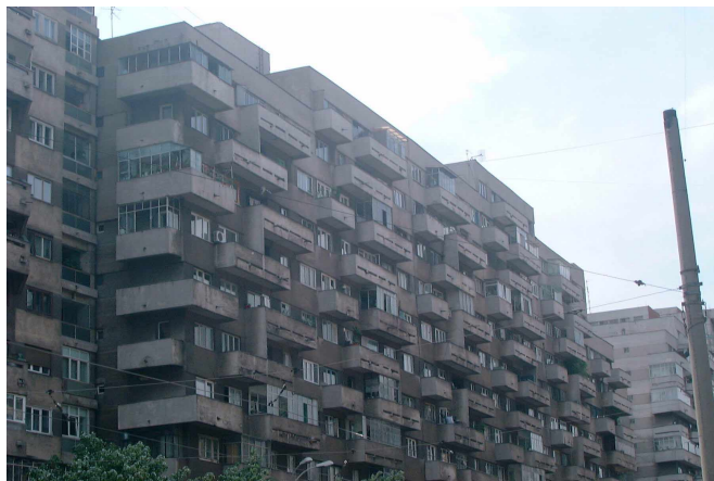
Fig.7 258, Pantelimon street (front view)
