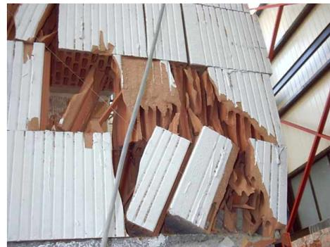
Fig. 12: Big horizontal movement in second floor's main wall (12 cm)
