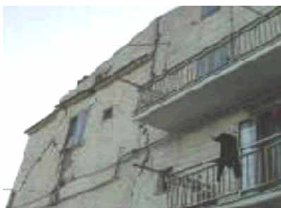
d) partial wall overturning
