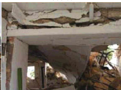
l) floor beams pulling out from the vertical wall
