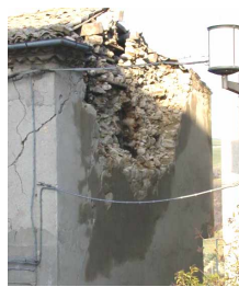
f) wall flexural failure
