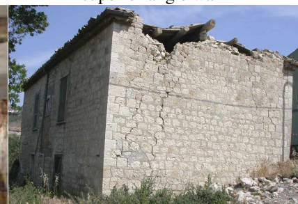
q) roof wall belt out-of plane overturning
