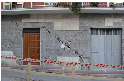
a) in-plane shear actions
