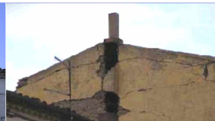
n) material irregularity, local weakness, etc.
