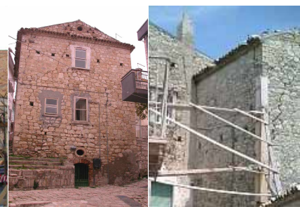
p) out-of-plane overturning of the superior angle wall
