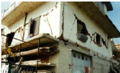
b) in-plane shear actions in the higher wall belt
