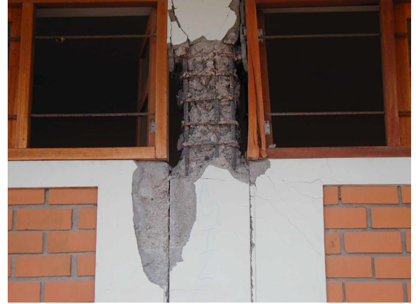
Figure 10. Damage to building designed using 1977 Standard.
