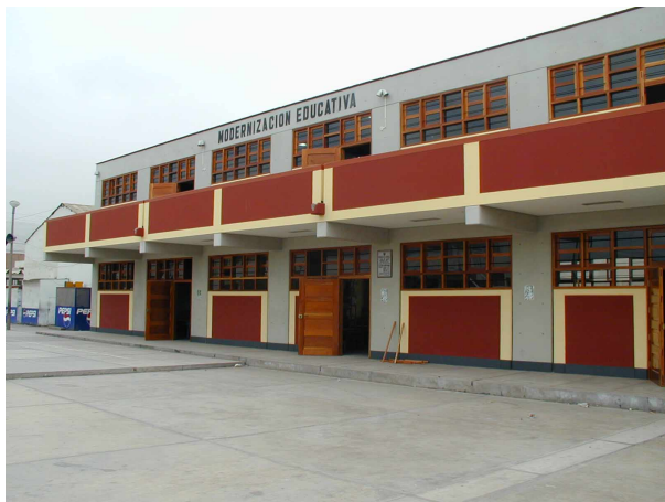
Figure 11. Post earthquake condition of school building designed using 1997 Standard.
