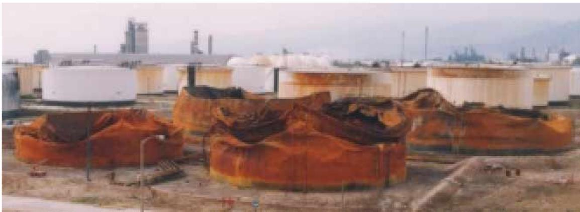
**Figure 4: Floating roof tanks destroyed by a huge fire**
