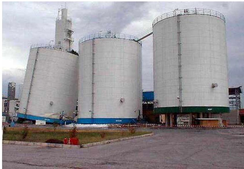
**Figure 7: Failure of the concrete pillar support of two cryogenic liquid oxygen tanks.**
