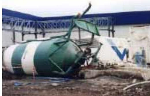
**Figure 6: Buckling of the supporting legs**
