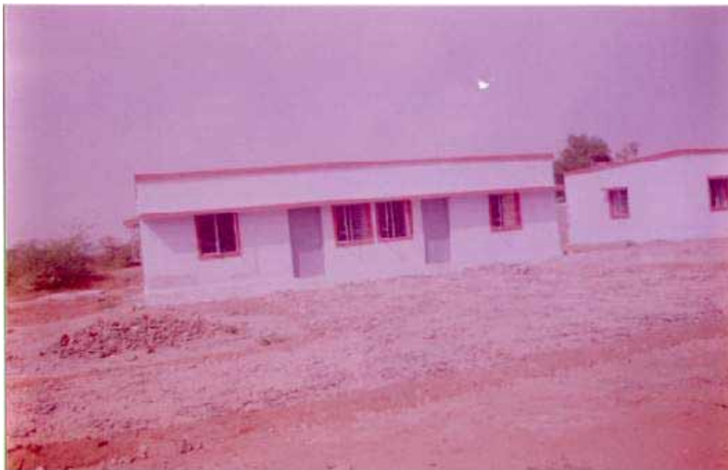
Photo no.3: Intact Single Storied Load Bearing Structure of Railway quarters At Aundh, 20 km from epicenter
