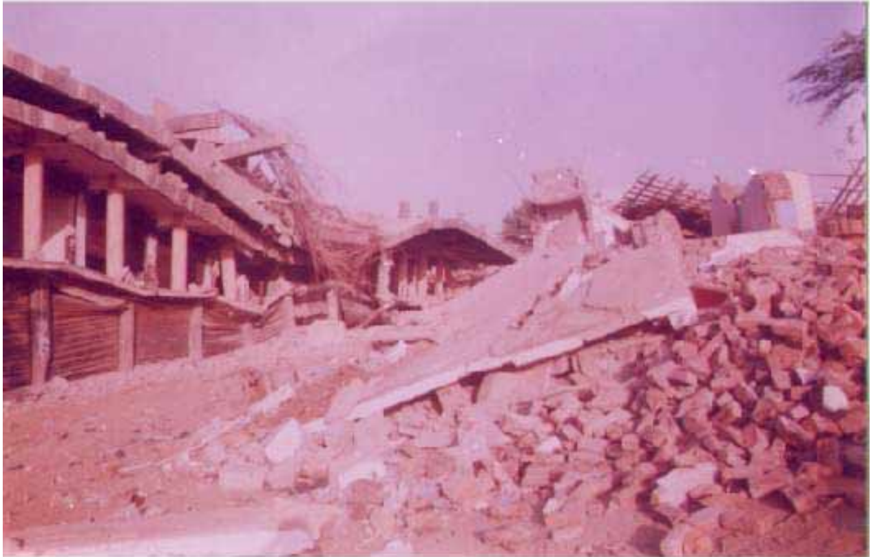
Photo No. 4 : Total Collapse Of Framed Structure At Bachau
