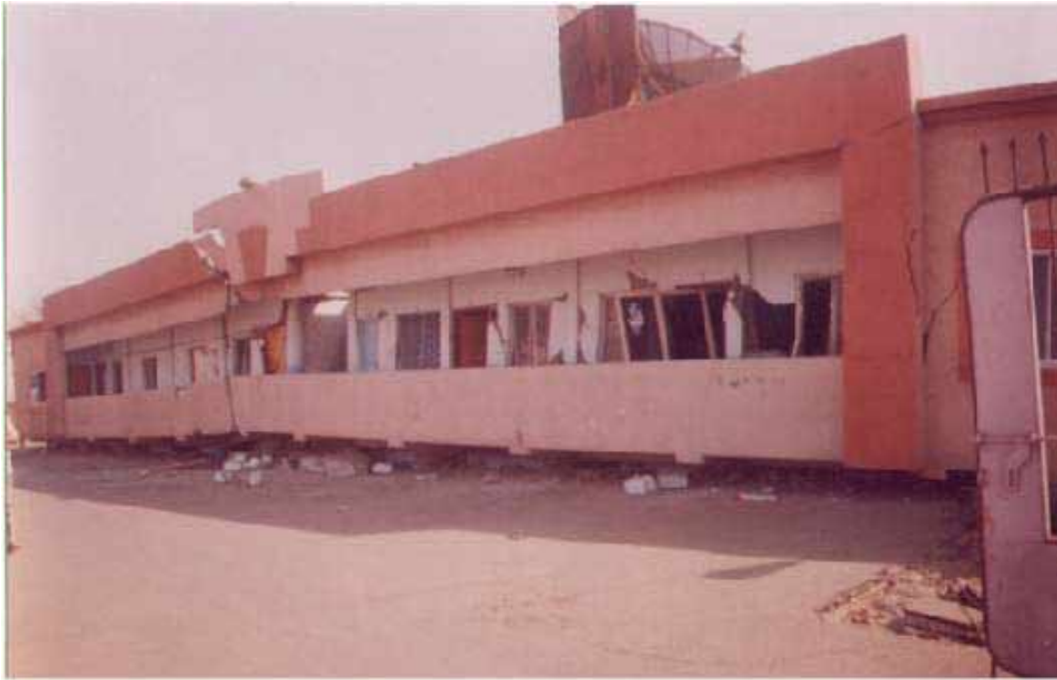
Photo No. 8 : The First Floor Looks Like Ground Floor (Hostel At Kandala Port )
