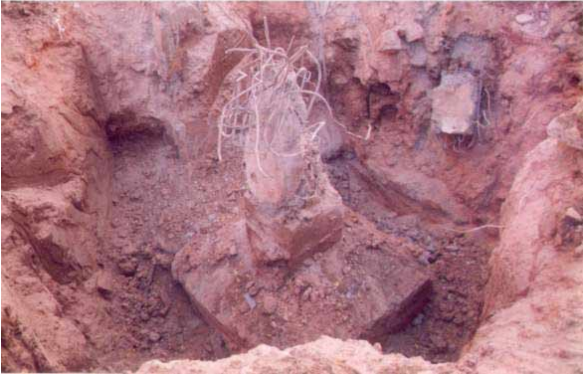
Photo No. 7: Exposed footing and column of framed Structure At Ahmedabad (Shikhar tower)
