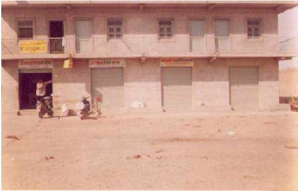
Photo No. 2 : Intact Two Storied Load Bearing Structure At Madhapur.
