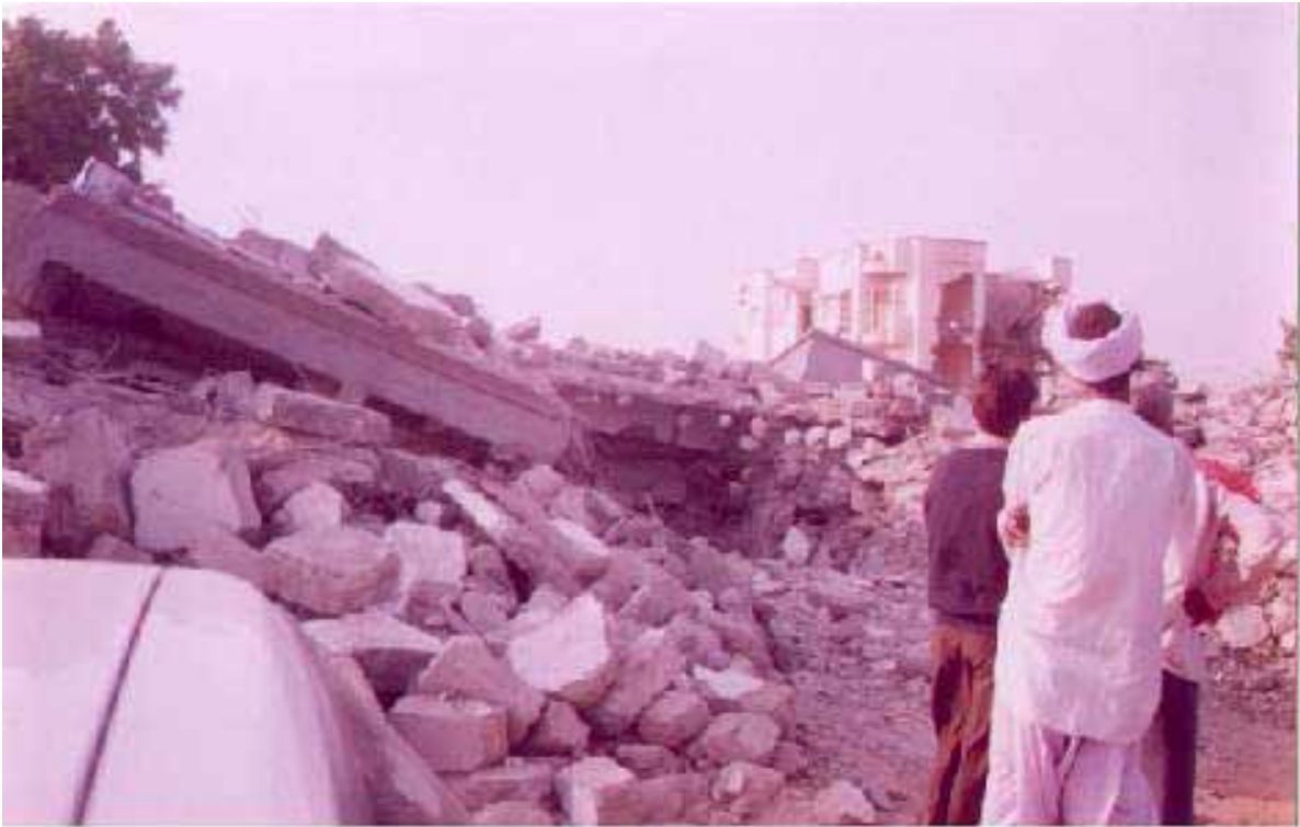
Photo No. 1 : Total Collapse at Bachau 18 Km. From Epicenter.
