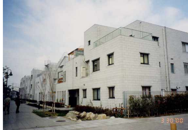
Fig. 2 A reinforced fully-grouted concrete masonry building in Japan
