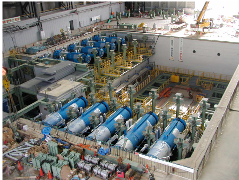
Figure 21: Installation of H-Actuator
