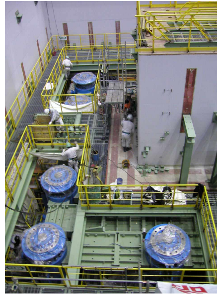
Figure 20: Installation of V-Actuators
