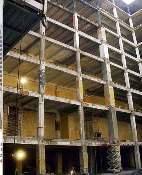
Figure 2. Eaton Building – View from atrium during construction.
