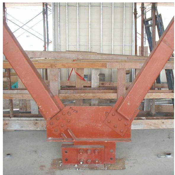
Friction damper in chevron bracing (inverted)
