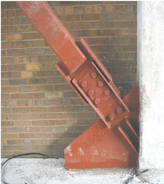
Friction damper in single diagonal bracing
