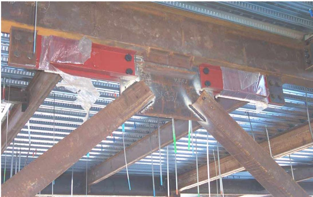
Figure 5. Typical Chevron brace with two friction dampers at the apex (during construction)
