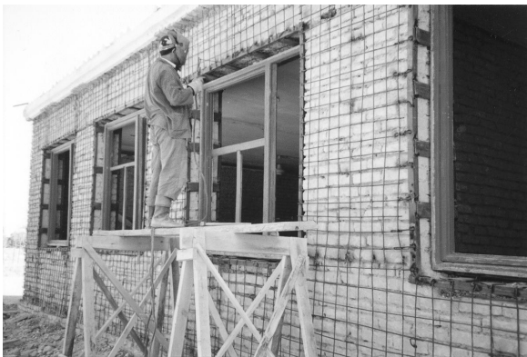
Figure 14. Strengthening measures – ductile shells and steel enframed windows [4].
