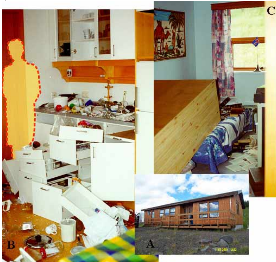
Figure 2: An earthquake-resistant residential building in the June 17th 2000 earthquake area (distance to fault 3,4 km). Photo A: The residential building from outside. Photo B: The victim's position inside (inserted figure) during the earthquake (MMI VIII). Photo C: A bookcase had fallen on the bed when the resident was absent (same building).
