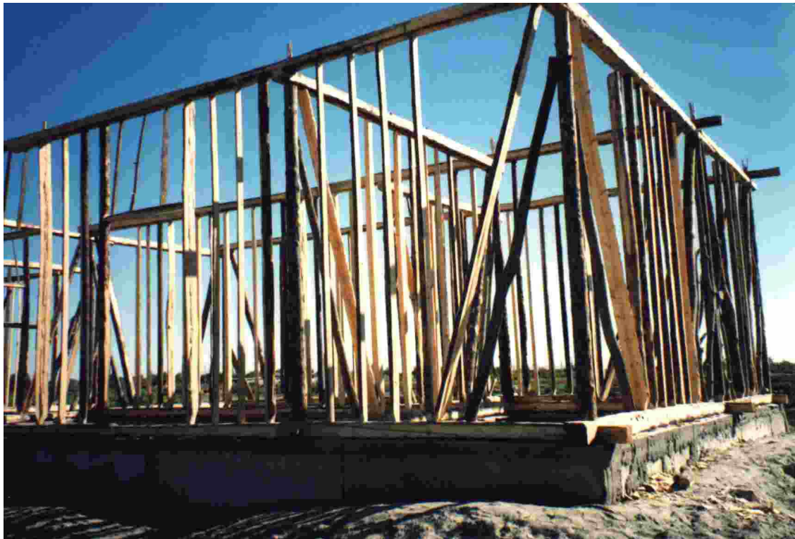
Fig.2. General view of construction of wooden frame (synch) house in Bukhara district, Uzbekistan
