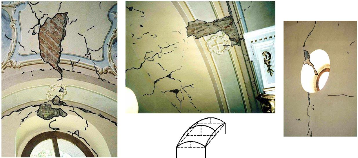
**Figure 6. Damage to Jasenov orthodox church Prussian vault**
