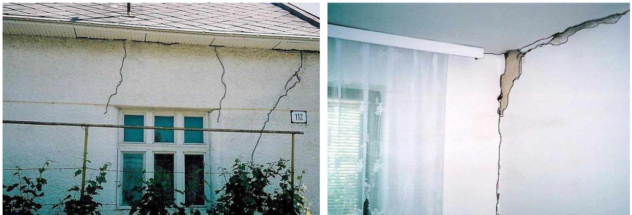
**Figure 7. Typical cracks in solid brick masonry of family house in Jasenov**
