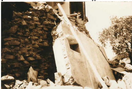
Fig. 5: Bachau Station Building showing the condition of a reinforced concrete column provided in masonry building.
