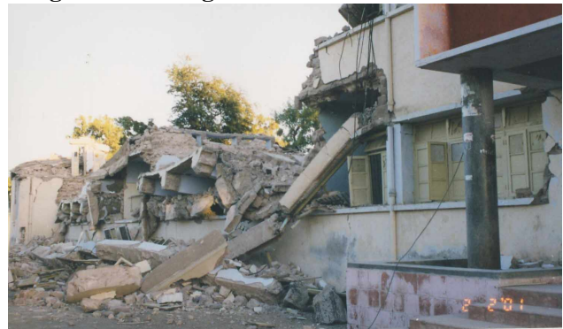
Fig. 4: Collapsed two story college building had linear plan with too many openings in front.
