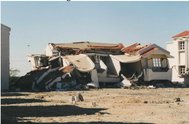
Fig. 1: Collapsed building built on drain side. Retaining wall at back also failed
