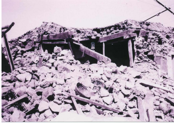
Fig. 9: In Killari in 1993 many traditional buildings with vertical timber frame inside survived the earthquake even with heavy roofs. Newly built houses without timber frame but with similar heavy roof of timber and earth were razed to ground.
