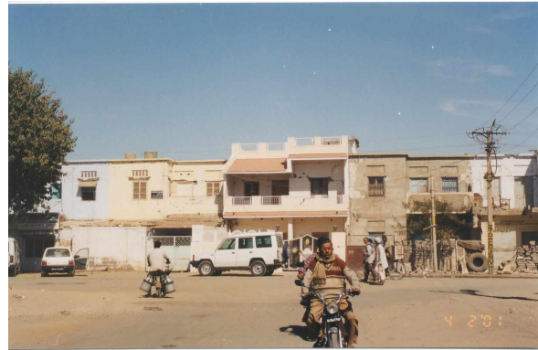
Fig. 12: At Gandhidham in this complex of well built row houses made of reinforced hollow block masonry, minor damage occurred only in the renovated house.
