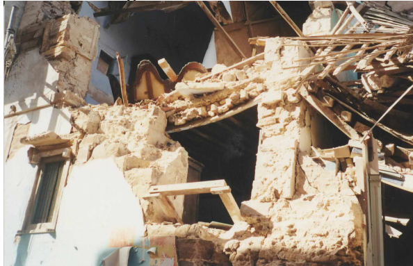
Fig. 11: In urban area attic of traditional house shown in Fig. 10 was converted into living space. Later traditional roof must have been replaced by concrete slabs. Such buildings killed many persons in Bhuj.
