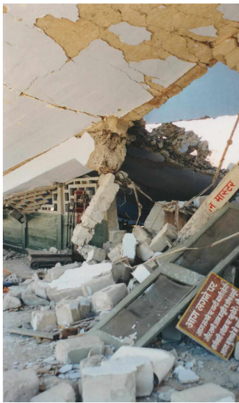
Fig. 5: Bachau Station Building showing the condition of a reinforced concrete column provided in masonry building.
