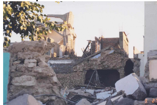
Fig. 6: In Chamoli Earthquake, column raised on the top of the stone wall slipped from its place due to lack of connection.
