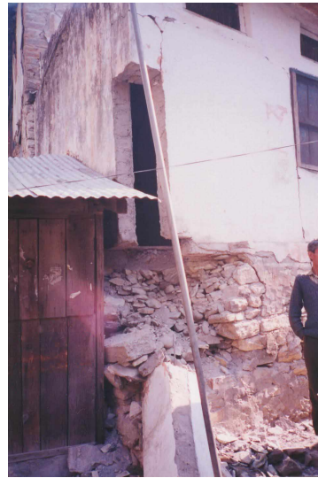
Fig. 6: In Chamoli Earthquake, column raised on the top of the stone wall slipped from its place due to lack of connection.
