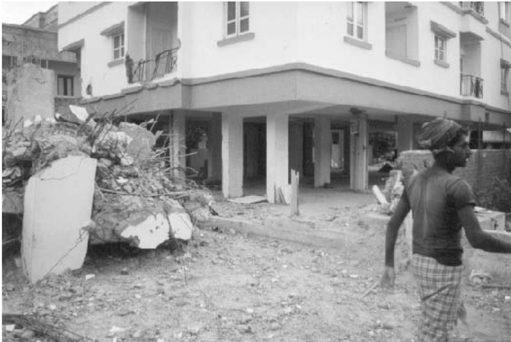
Photo No 7 Frame Structure With Flexible Ground Floor.
