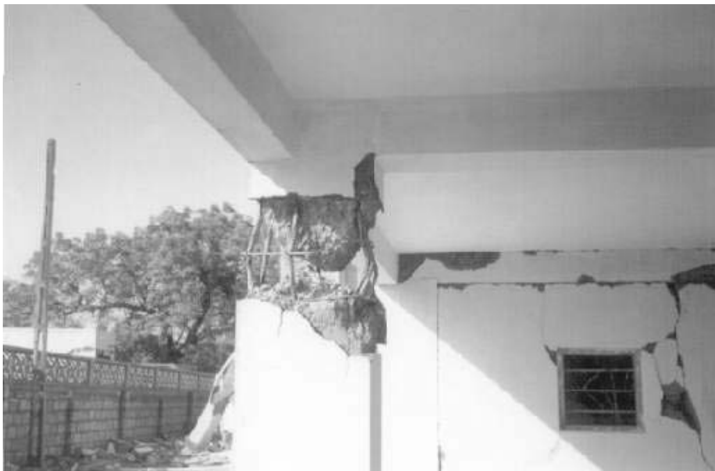
Photo No 8 Failure Of Ground Floor Column
