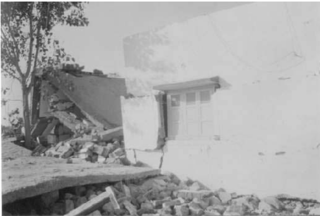
Photo No 2 Partially Damaged Load Bearing Building Another View
