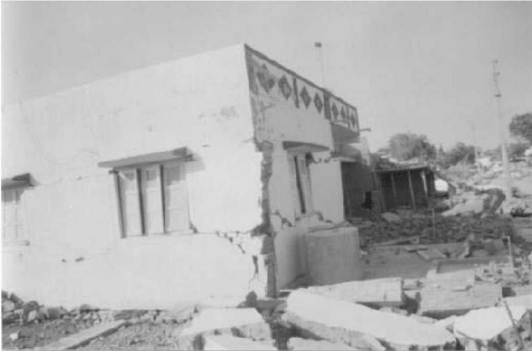
Photo No 1 Partially Damaged Load Bearing Building
