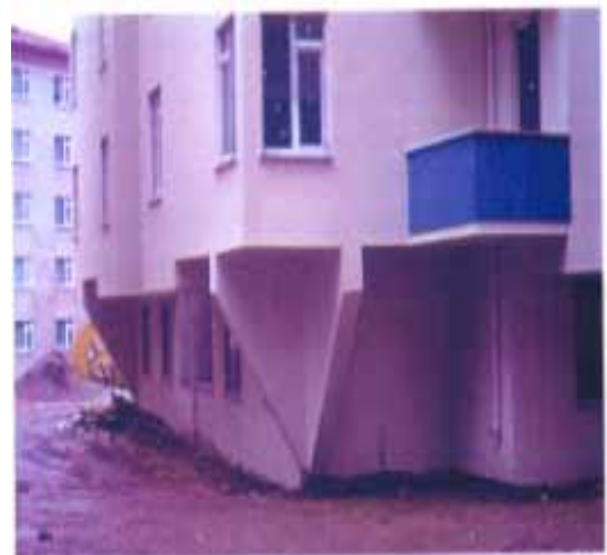
Figure 2 General views of two buildings having second kind consoles
