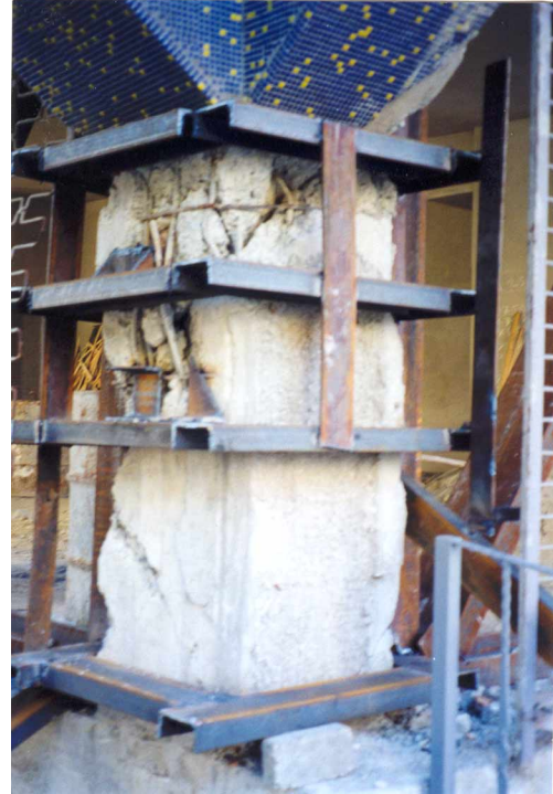
Figure 7 Corner columns damaged heavily connected corbels in two directions (shear failure)
