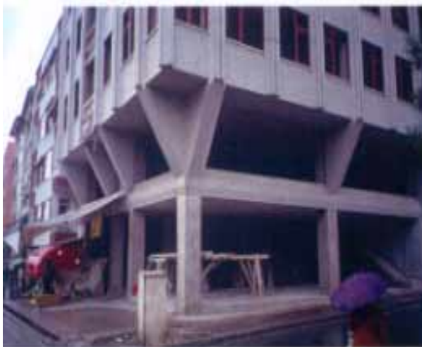
Figure 2 General views of two buildings having second kind consoles
