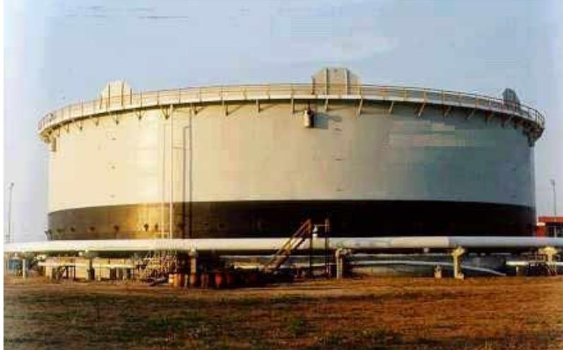
Figure 3 – Circular cylindrical steel storage tanks of 200 thousands barrels
