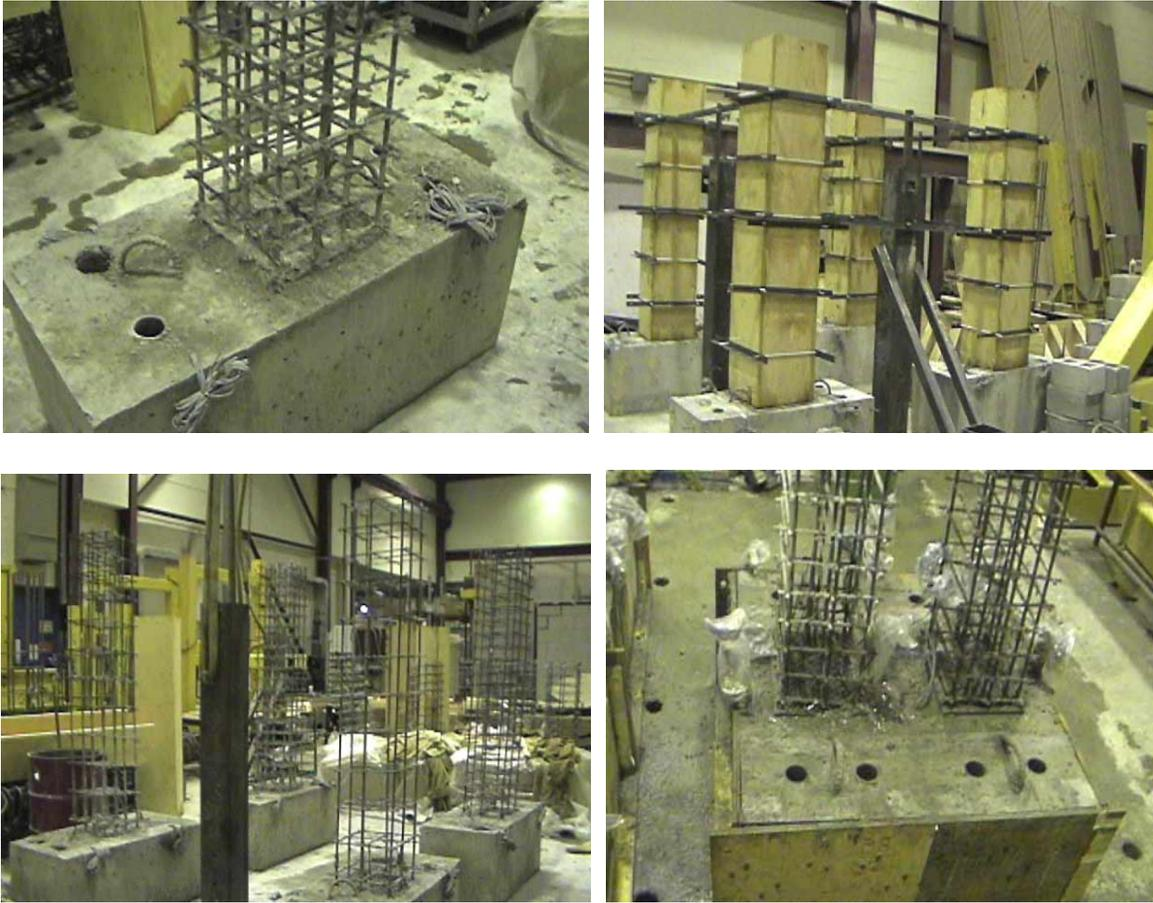
**Figure 5 Views of column and beam cages and the two stage casting process employed**
