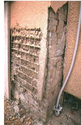
Fig. 3: Loss of effectiveness of a wall strengthened with jacketing due to the scarce connection of the steel net through the masonry and the lack of overlapping of the reinforcement at the corners.
