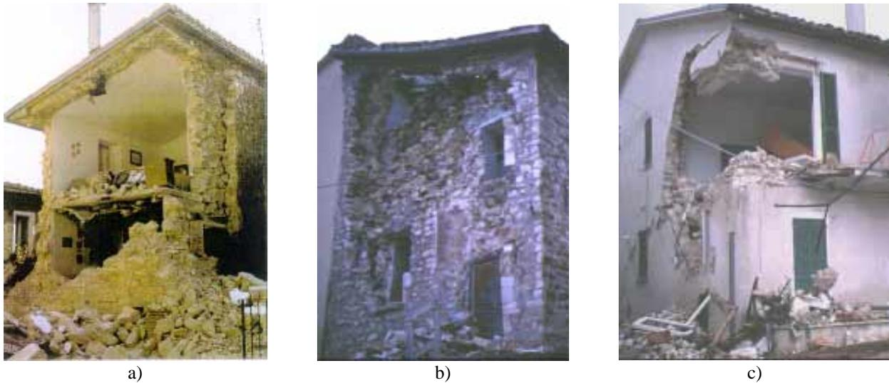
Figure 4: Out-of-plane mechanisms on existing building under seismic actions: collapse of the façade due to the lack of connection between floors and wall and among walls (a), expulsion of the external layer of the wall due to the multi-layer poorly connected constructive system (b), collapse of the corner due to the excessive nearness of the openings (c).
