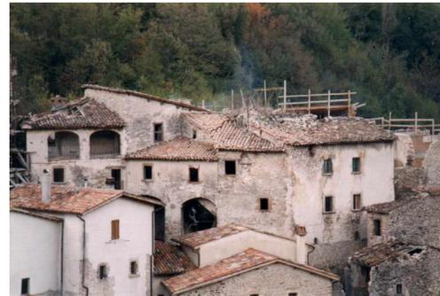
Fig. 16: View of the units named RcC9, RcC10, RcC5 and RcC4 with evidence of damage on masonry walls and roofs.
