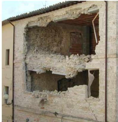
Fig. 2: Rear of the same building where a large overturning of the façade occurred, due to the high percentage of openings, combined with the presence of a heavy r.c. floor supported by a single layer of the poorly connected double-layer masonry.
