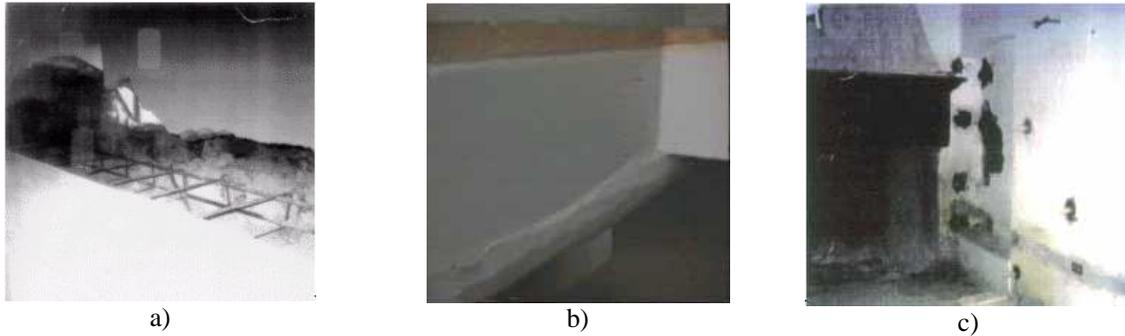
Figure 10: Interventions performed before the last earthquake on floors (a: execution of the r.c. tie-beam, b: detail of the r.c. floor) and walls (c: phase of injection) in the building located in Montesanto (Perugia, Italy).
