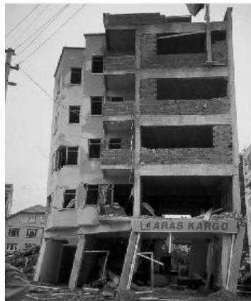
**Figure 2.** Effect of infills not uniformly distributed in height for a building under seismic action
