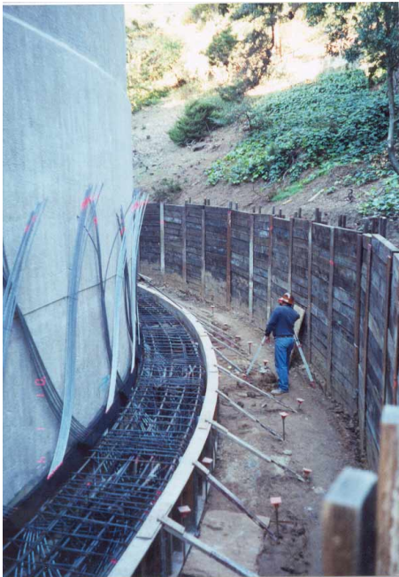
Figure 4. Exterior Seismic Cables & Ring Footing Addition
