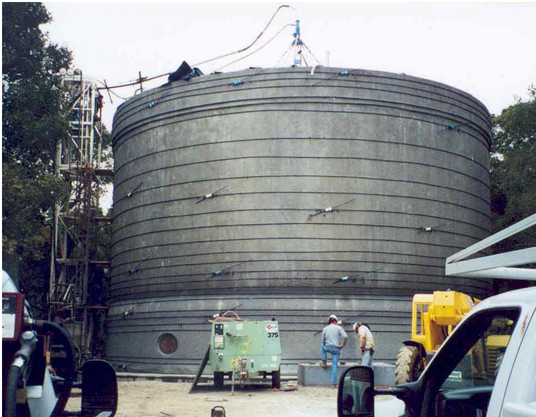
Figure 6. Post-tensioned Tendons prior to final shotcreting (Note: bottom of wall has new seismic cables that are encased in new shotcrete)
