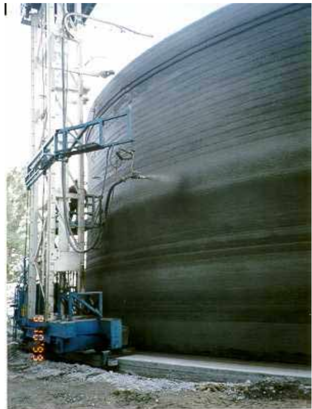
Figure 5. Automated Wire or Strand Wrapping and Shotcrete
