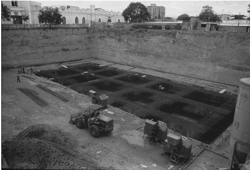
Fig. 7. Reinforcing steel of rectangular mat.
