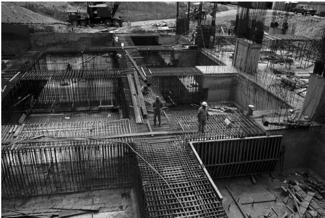
Fig. 10. Construction advancement square mat. Note inverted shear-key joints. Building 60 meters high.
