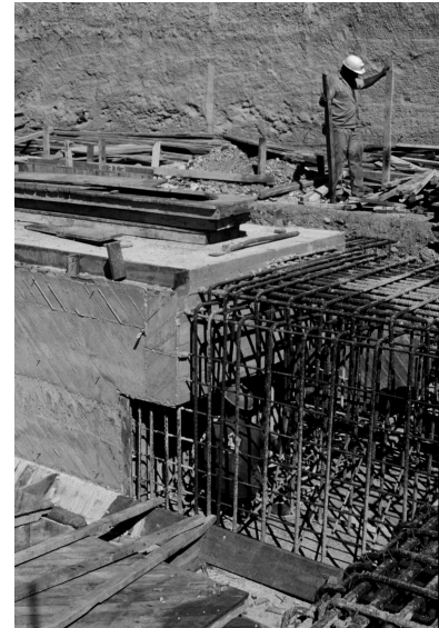
Fig. 8. Detail of inverted shear-key joint.
