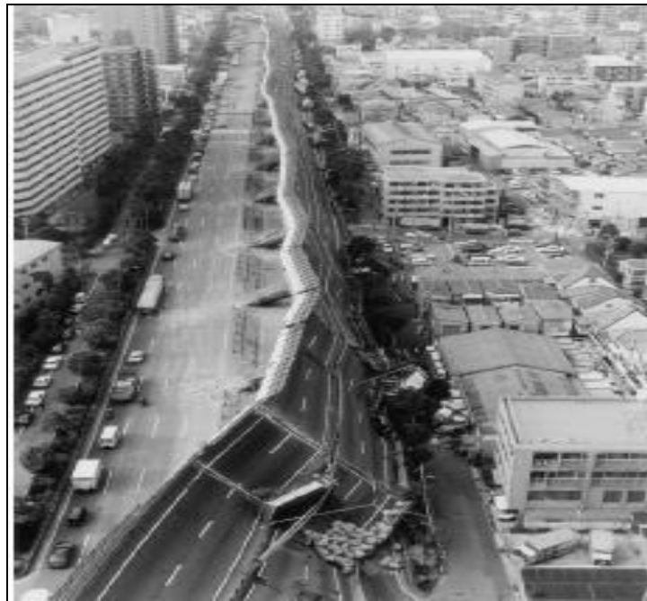
Figure 1 Collapse of elevated bridges in 1995 Kobe earthquake
