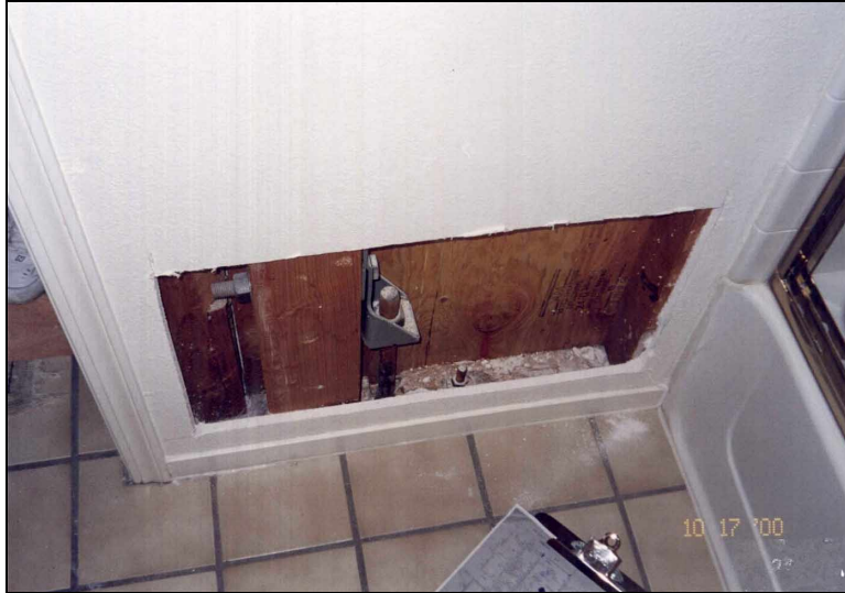
Figure 3: This holddown is inset by more than 12-inches.
