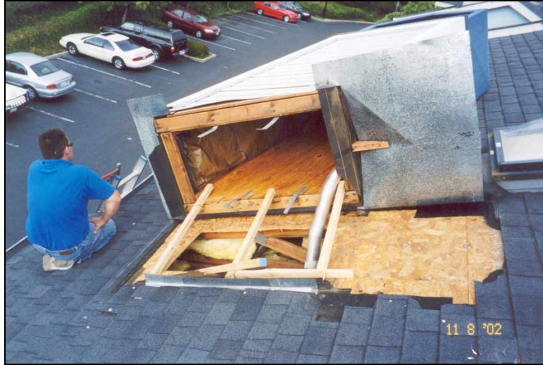
Figure 6: This chimney collapsed during a wind storm due to the contractor's failure to nail the bottom halves of the holddown straps.
