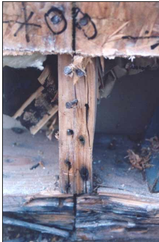
Figure 2: Nails were installed too close together at this stud, causing the stud to split.
