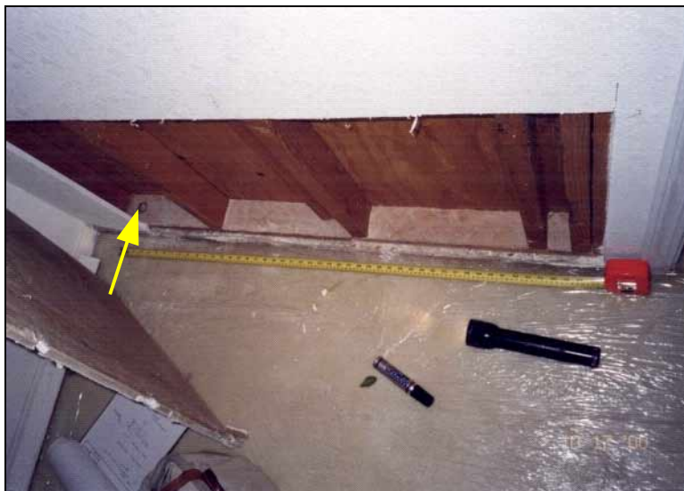
Figure 8: This sole plate only had one nail (yellow arrow) in 48-inches.
