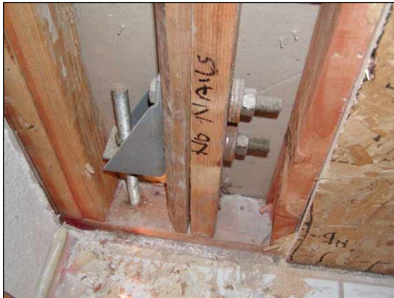
Figure 4: This holddown was inset; the holddown studs were not internally nailed; and the plywood was not nailed to the holddown studs.
