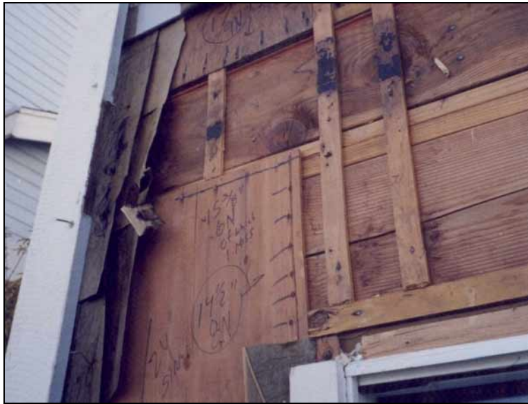
Figure 9: The second floor plywood was nailed to the second floor sole plate and the first floor plywood was nailed to the first floor double top plate, resulting in a discontinuous load path. Furthermore, the first floor plywood nails were installed between the plates of the double top plate, resulting in a connection with little or no capacity.
