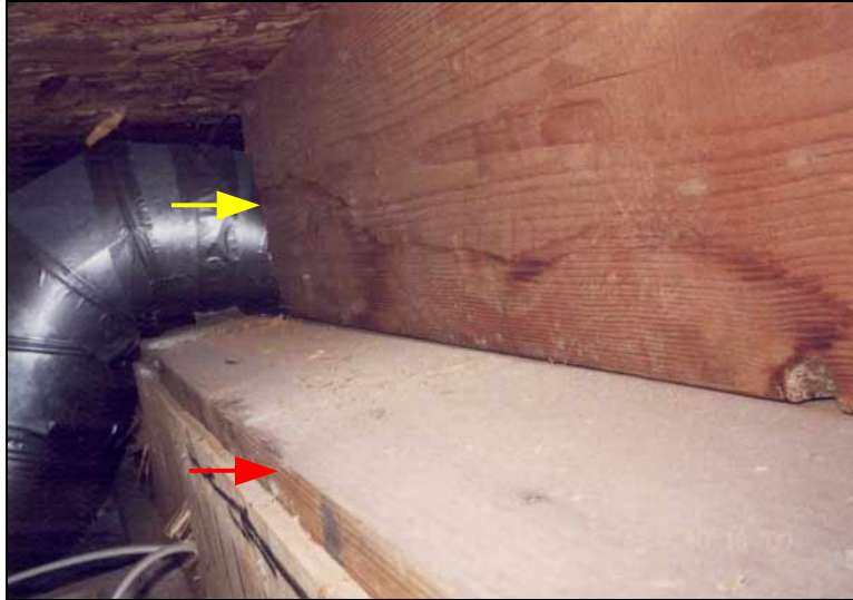
Figure 7: The required clips from the rim joist (yellow arrow) to the double top plate (red arrow) were not installed.
