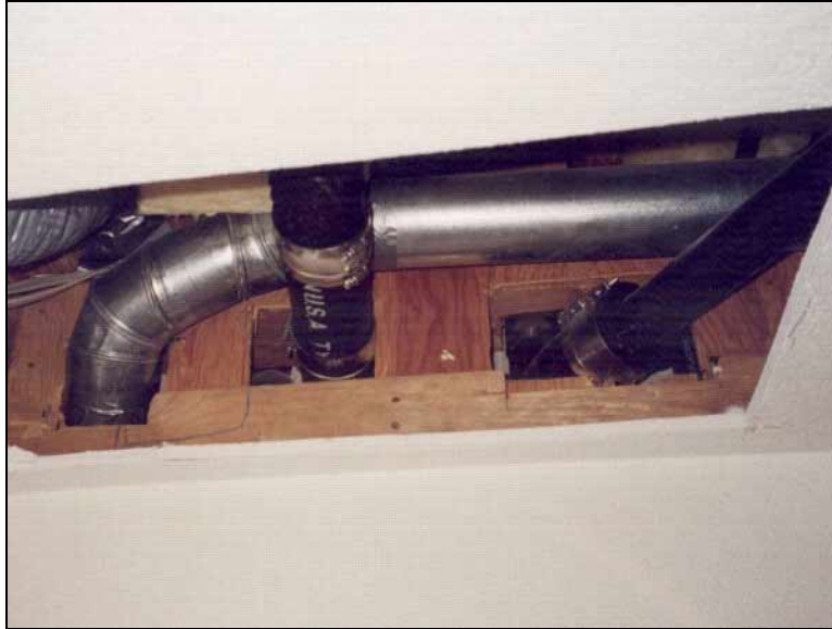
Figure 10: This plywood shear wall is severely compromised by the HVAC and plumbing installation.
