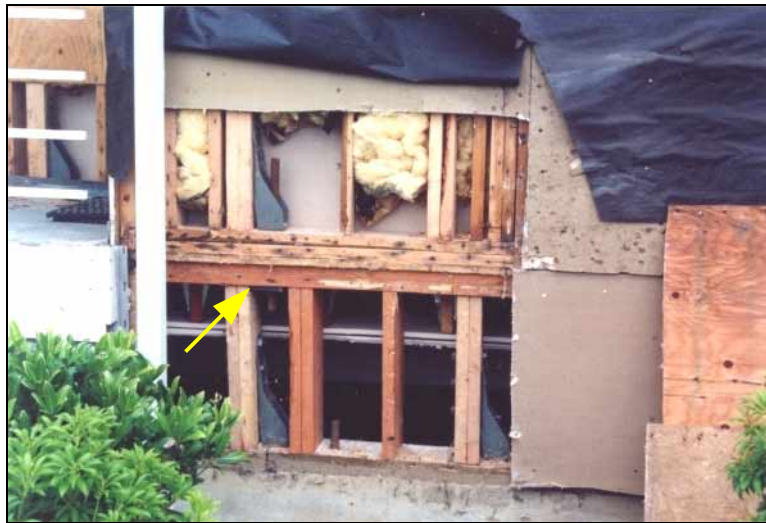
Figure 5: The holddown on the first floor is not connected to anything but a plate washer on the underside of the double top plate of the crawlspace (yellow arrow), resulting in a discontinuous load path.
