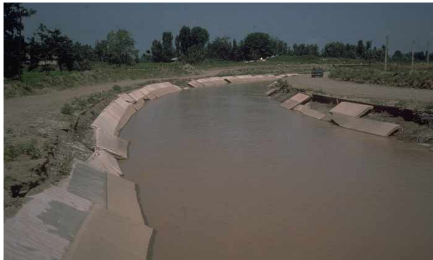
Fig. 5: Irrigation canal lining damaged during the June 21, 1990 Manjil earthquake in Iran (rigid body movement of concrete elements)
