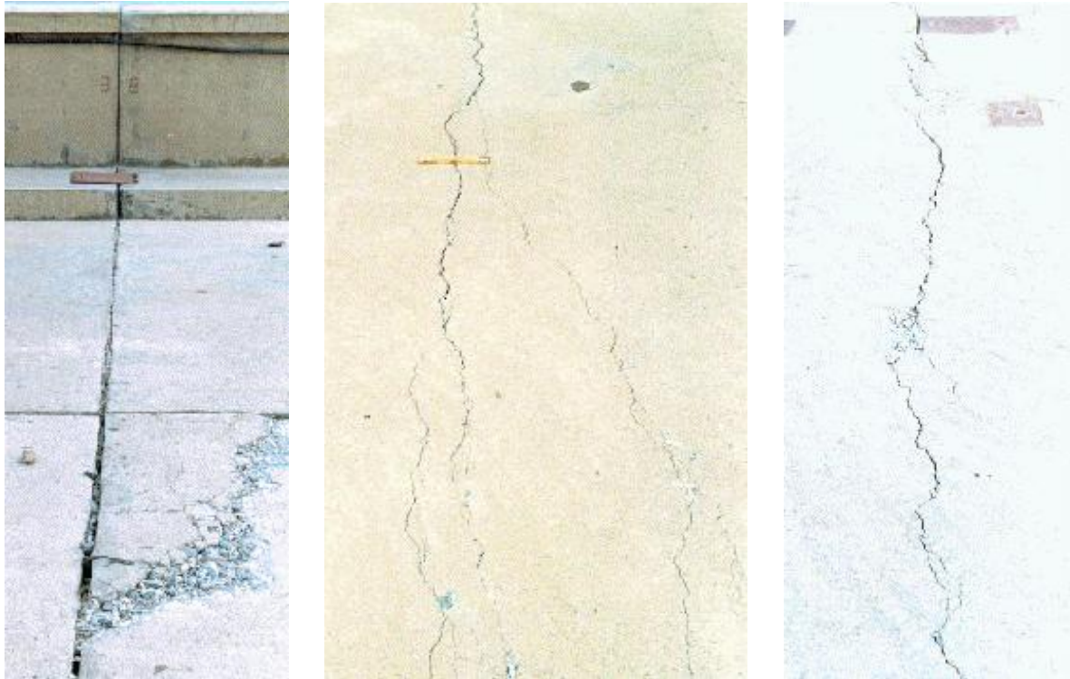
Fig. 6: Cracks at the crest of the 106 m high Sefid Rud buttress dam, caused by the June 21, 1990 Manjil earthquake in the Alborz mountain range in the Northwest of Iran. Left hand picture: local compression failure of deck slab at joint of two adjacent monoliths; central and right hand pictures: cracks on concrete slab on dam crest in direction of dam axis on different blocks (note: cracks shown are caused by the cross-canyon component of the ground shaking)
