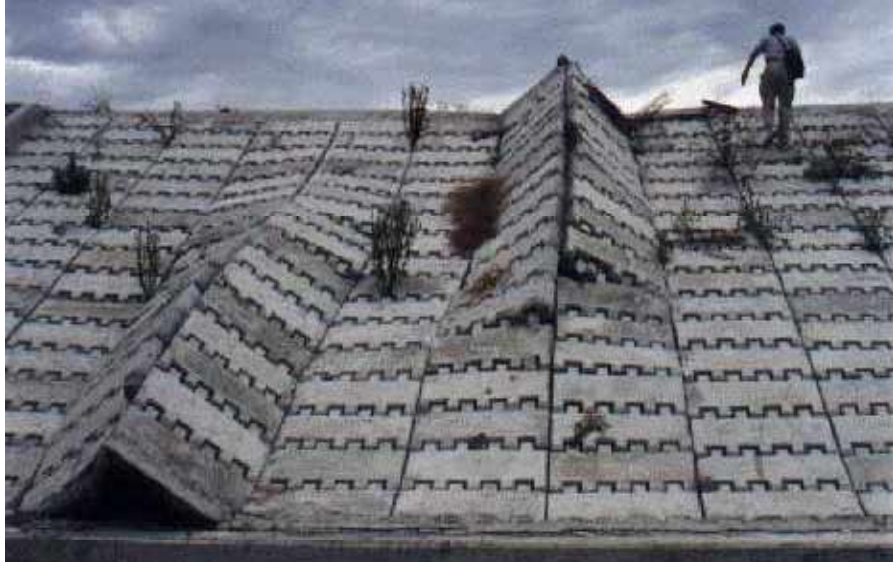
Fig. 4: Buckling of canal lining elements caused by the September 21, 1999 Chi-Chi earthquake in Taiwan
