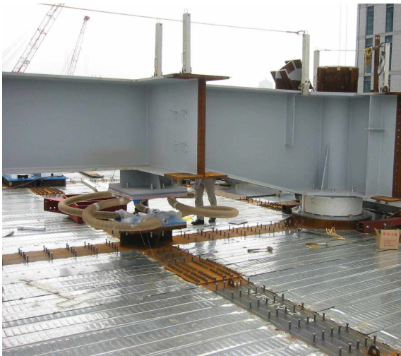
Photo.2 Construction of Isolation Interface
