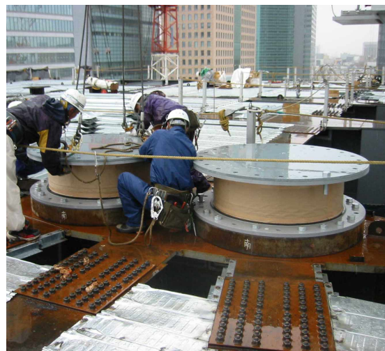
Photo.2 Construction of Isolation Interface
