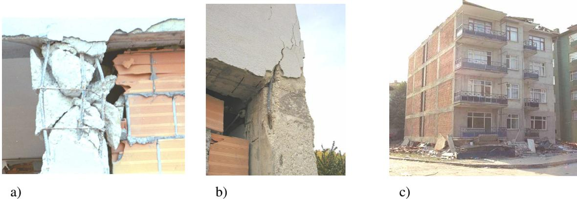
**Figure 1 Observed effects of interaction between infills and bare frame: a) shear failure of column and b) exterior joint shear damage (Bonafro, Molise 2002); c) global collapse for soft storey mechanism (Izmit, 1999, NISEE image collection)**
