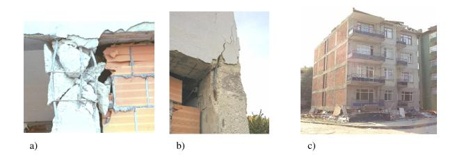
Figure 1 Observed effects of interaction between infills and bare frame: a) shear failure of column and b) exterior joint shear damage (Bonefro, Molise 2002); c) global collapse for soft storey mechanism (Izmit, 1999, NISEE image collection)
